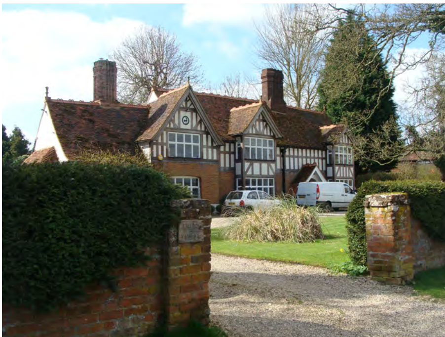
Picture 1.8 Croys Grange an impressive building near the River Chelmer whose front is 19th century with imitation timber framing.
