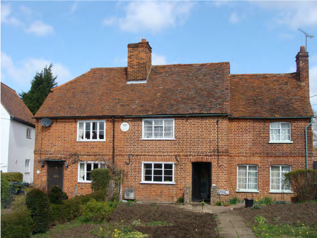
Picture 1.18 Hillside Cottage, a quality 19th century red brick building with centrally located circular plaque displaying letter M of the Maynard family.
